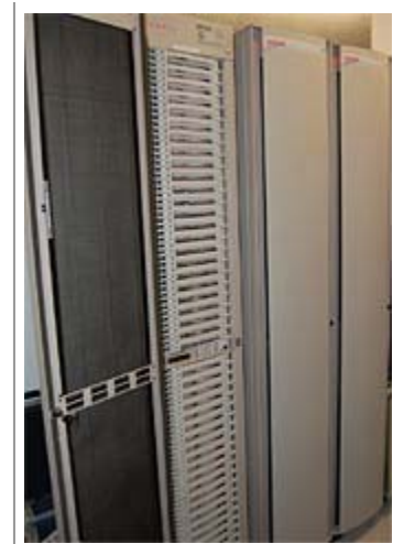
Figure 1: Centralized dimming places all the dimmers together in a rack system, such as this ETC Sensor dimming rack. Photo courtesy ETC.
