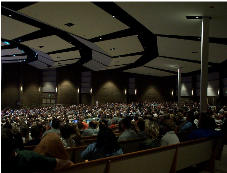
Crossroads Community Church in Vancouver, Washington was designed with "V" shaped ceiling clouds. The front facing surface of the clouds is covered with sound absorbing materials to help control the sound from the speaker systems. The rear facing surface is made of drywall to reflect congregational singing sound back into the seating area.
