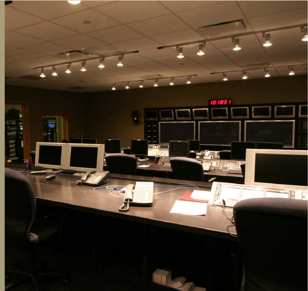
Video production control is located downstairs in the facility. At the front of the room is a large videowall made up of both LCD and plasma screens. The router can put any source or any camera on any monitor giving flexibility to the variety of video directors.
